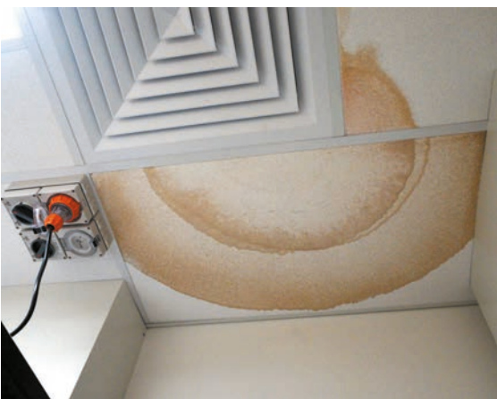
Water intrusion through the roof space was obvious.
