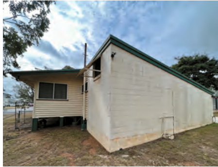
Blackbutt Station was described in Parliament as decrepit, tiny and not functional. The QPU wants authorised upgrades to Blackbutt to be expedited.
