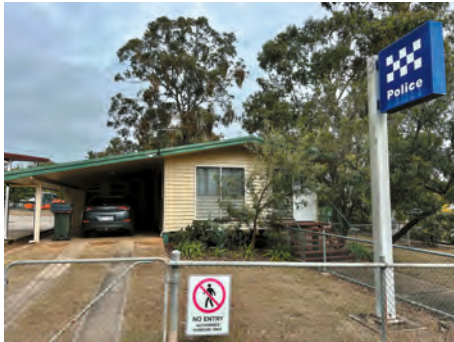
The Blackbutt Police Station faces the D'Aguilar Highway on the Southern side of the township.
