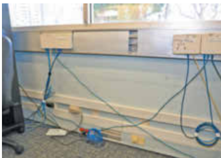
Open exposed cabling in the desk area in the Maroochydore Station day room.
