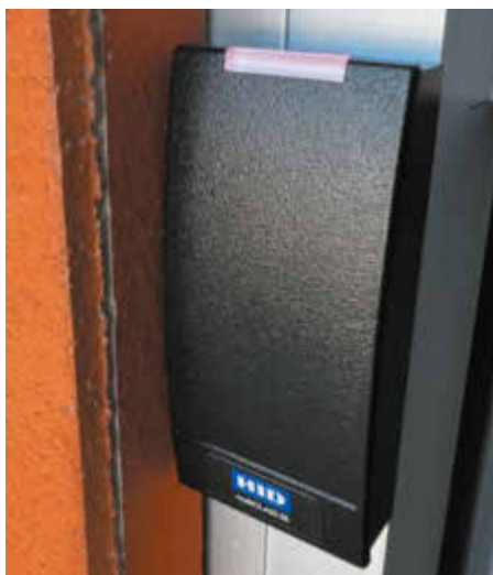
The plan is for all exterior doors and internal security areas to be fitted with fob readers to allow fast secure entry and monitoring.
