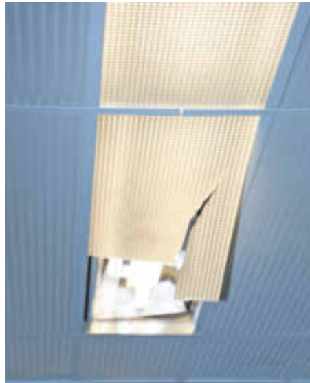
Damaged light fittings over the desk area in the day room potentially exposing officers below to dust and rodent waste.
