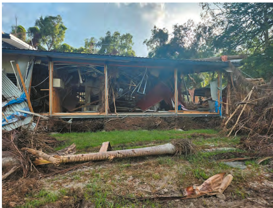
The floodwater blew out all walls on this property in Wujal Wujal.
