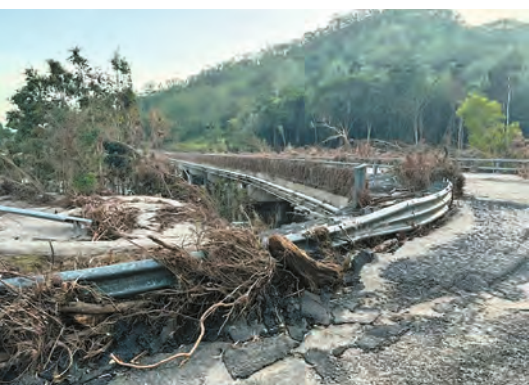
Bridges that did stay intact were covered in significant debris or roadways on each side were damaged.
