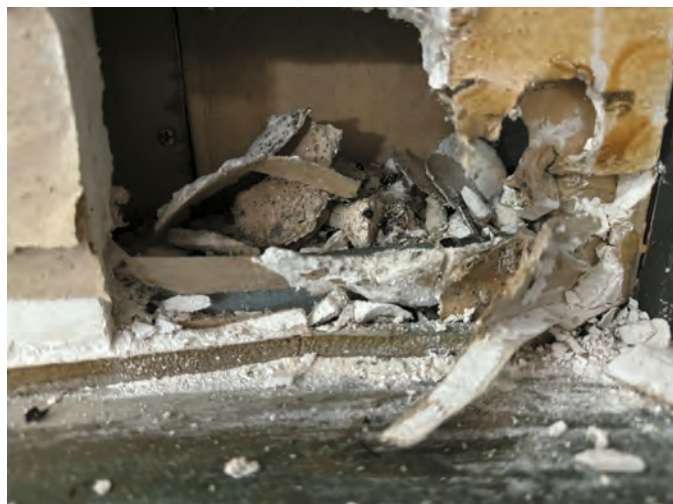
Inspection in every wall cavity revealed the presence of mould.
