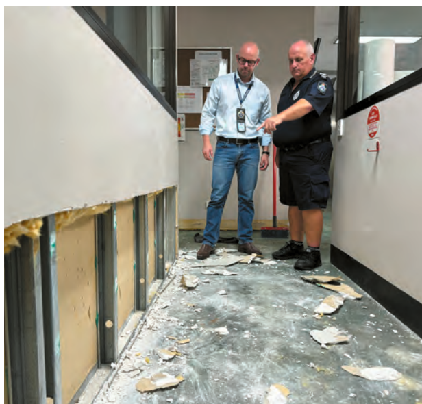
The initial work by QBuild was to cutaway the soaked gyprock but Sgt Smith explains to QPU Vice President Shane Prior that the entire sheeting will need to be replaced.
