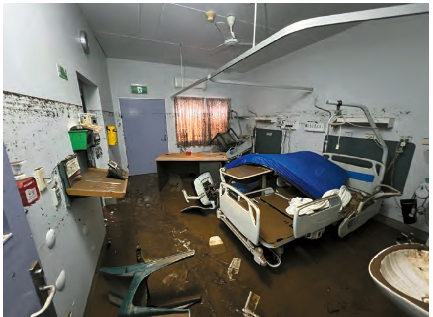
The Wujal Wujal clinic sustained significant damage from the initial floodwater surge and runoff. The high water marks are clearly visible on the walls.
