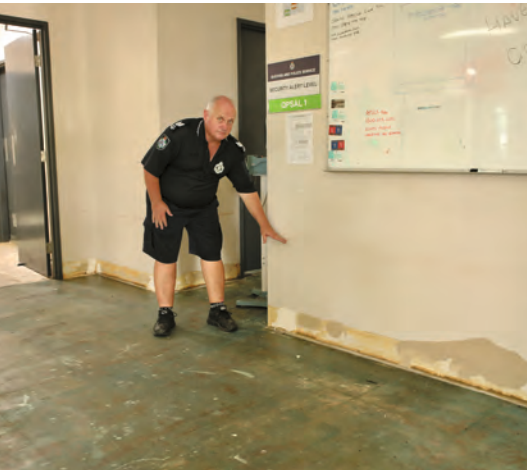
The water height inside the station. The damage was compounded by the presence of raw sewage from backflowing toilet drains.
