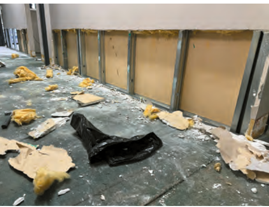
Some of the temporary strip out work completed by QBuild.
