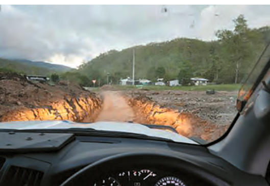
It took excavators hours to clear silt off the main street in Wujal Wujal and reach the original road surface.
