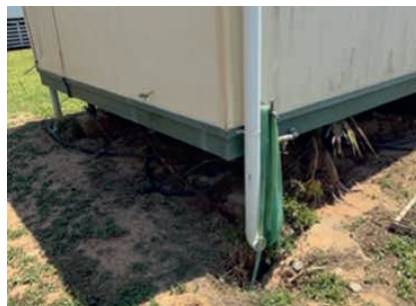
Drainage isn't connected, allowed to flow around building foundations and support structures.
