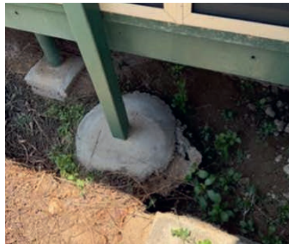
Support stumps are 'floating'.
